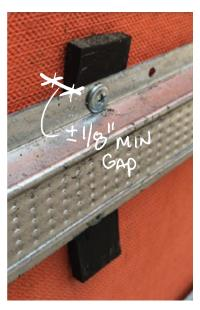
When we have an air barrier on the wall, sheet applied or liquid, any horizontal girt will need to be separated from the substrate or install sealant to repeal the moisture, to avoid moisture from resting on the wall, which will go through and damage the sheathing.
